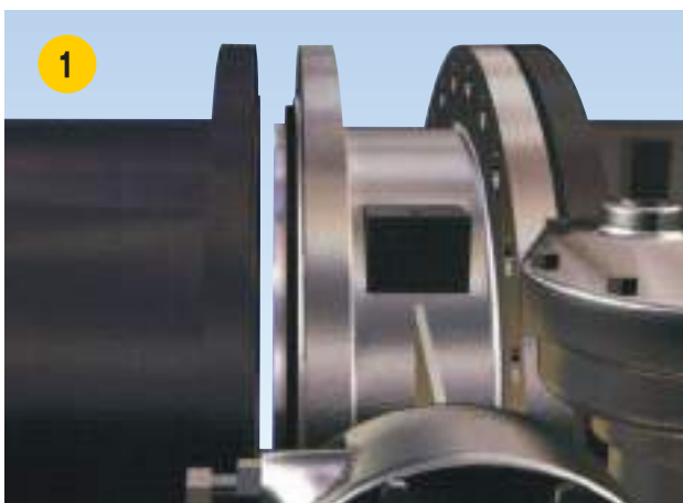
► Remove old valve and install Expansion Butterfly Valve
