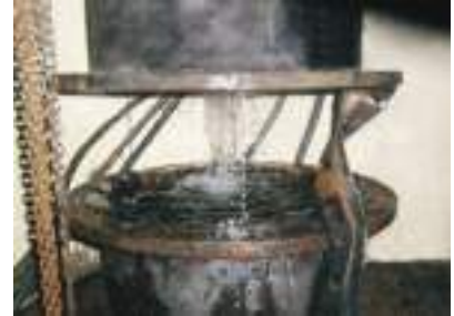
Removed(No damages on piping)
